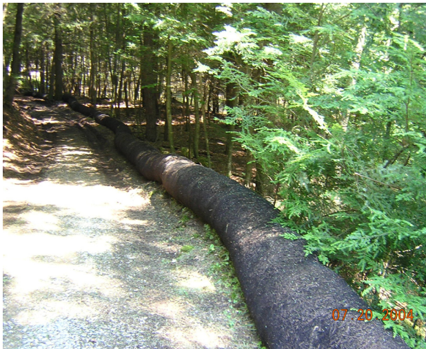
5 24 in Runoff Diversion Soxx™ for High Storm Flow
