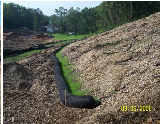
4 End Elevated Upslope to Prevent End Around Flow
