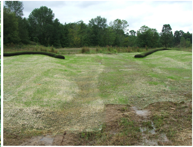
4 End Elevated Upslope to Prevent End Around Flow
